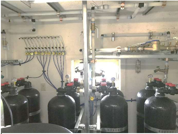
Exhibit 2-3: Portion of the [REDACTED] POET system. Sampling ports are shown in the upper left.
